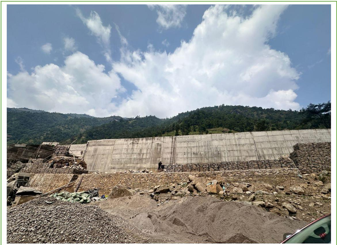
*Image 35: - Retention wall for backfilling at desander*
