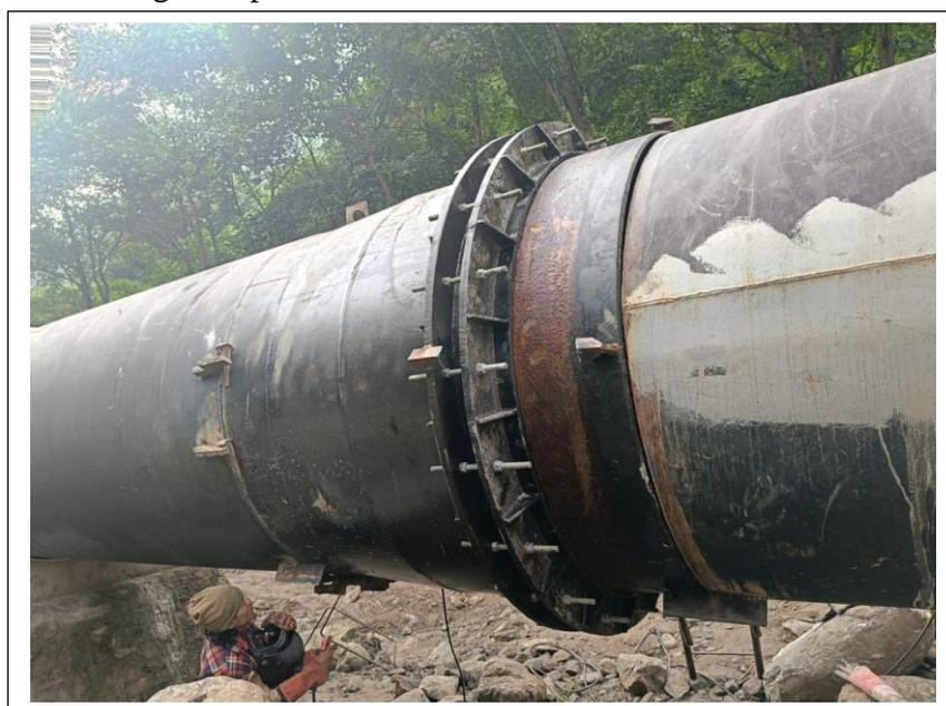
*Image23: Expansion Joint installation*
