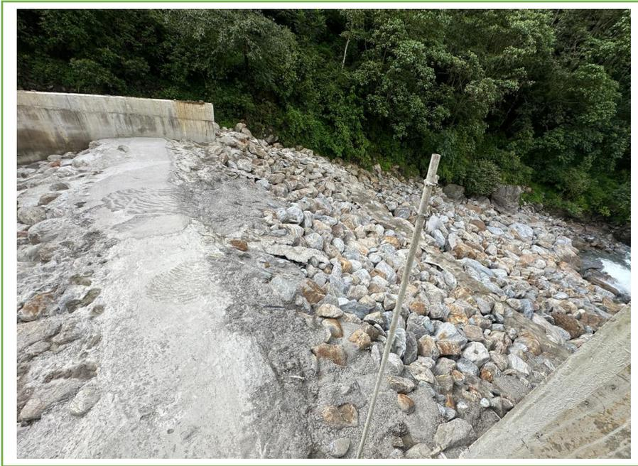
*Image 10: Boulder Riprap and concrete infill in weir*
