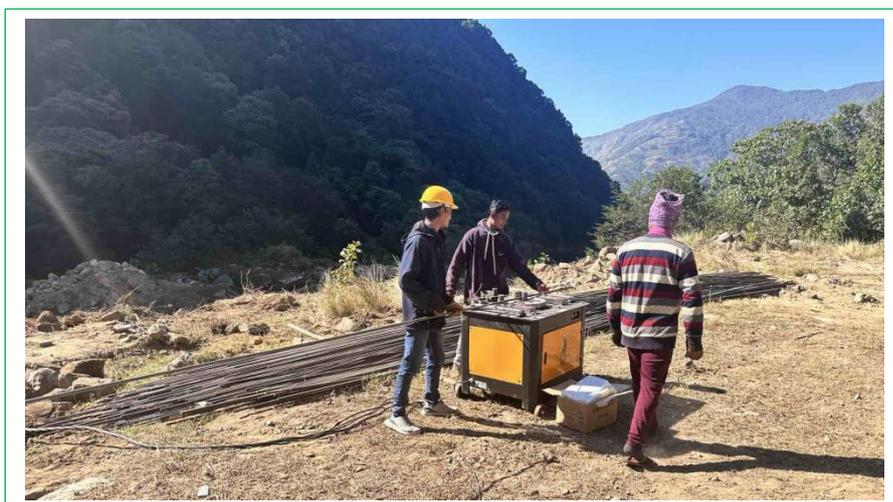
*Image 5: - Rebar Straightening and Cutting Yard*
