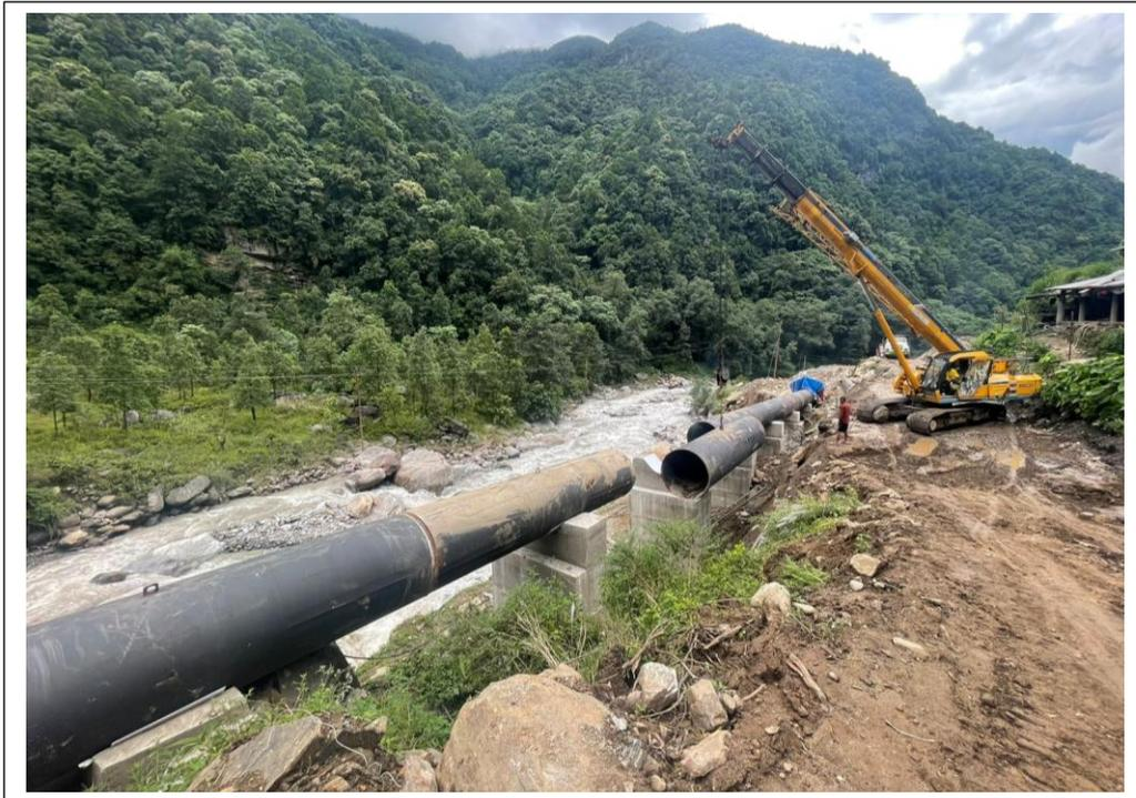
*Image22: Pipe erection in saddle support along AB 24-25*
