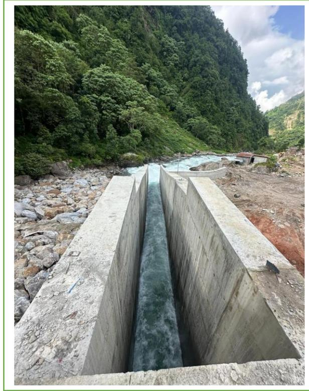
*Image 6: - River Diversion through Undersluice*
