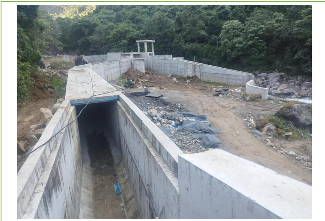
*Image 11: Approach Canal and undersluice wall*
