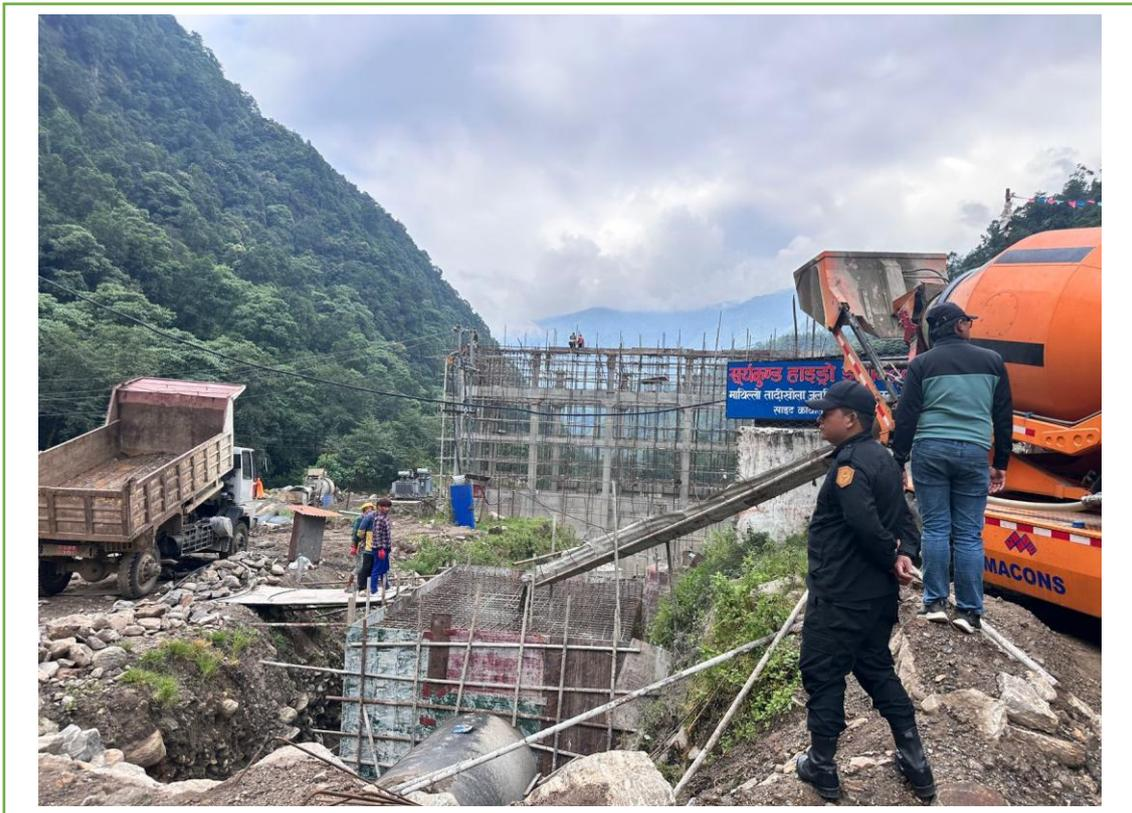
*Image 32: - AnchorBlock 26 Concreting*
