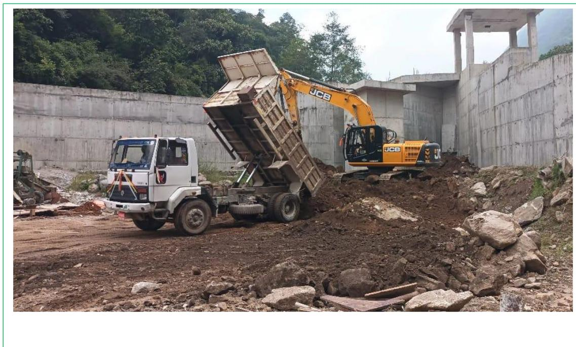
*Image 39: - Backfilling at intake*
