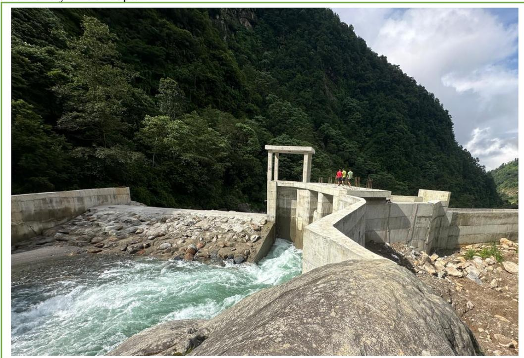
*Image 9: Weir and undersluice*
